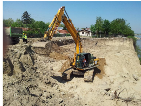
Fig. 2(b) Tracked excavator (bagger)
