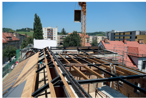
(b) Construction of a steel roof
