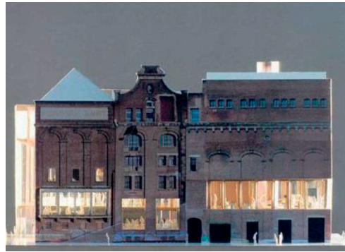
(b) After rehabilitation/reconstruction
