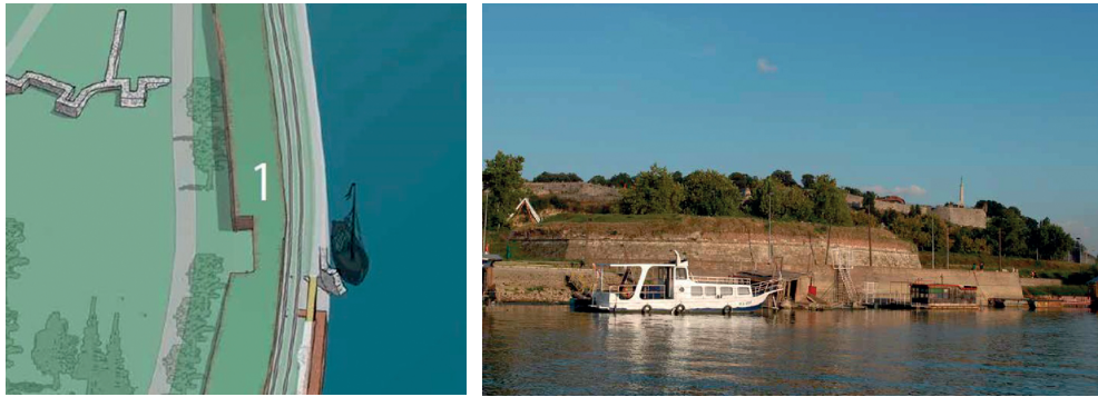
Figure 4.5. Riverside Rampart of Kalemegdan, © Institute for the Protection of Cultural Monuments of the City of Belgrade.
