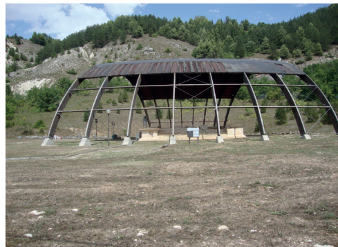
(b) The covering of the ancient temple in Castel di Ieri, L'Aquila, Abruzzo, Italy, originally located in a rural environment, re-proposes the monumental nature of the original structure, © L. Migliorati
