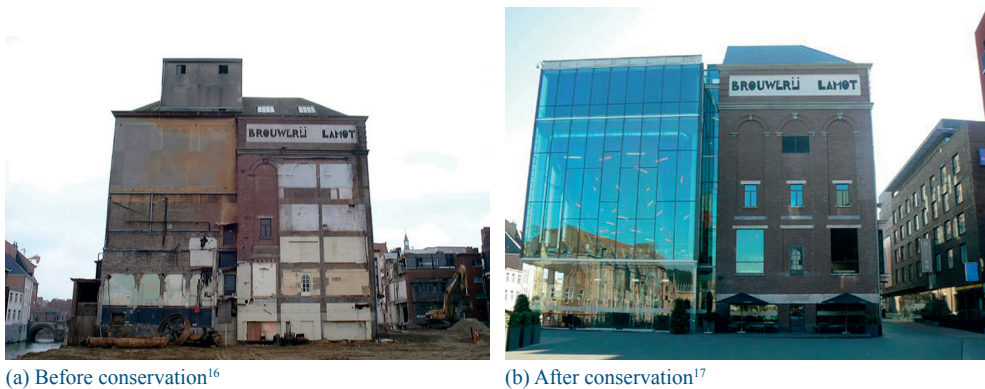
Figure 3.2. An example of a more drastic conservation approach used – Case 6 Lamot, BE.
