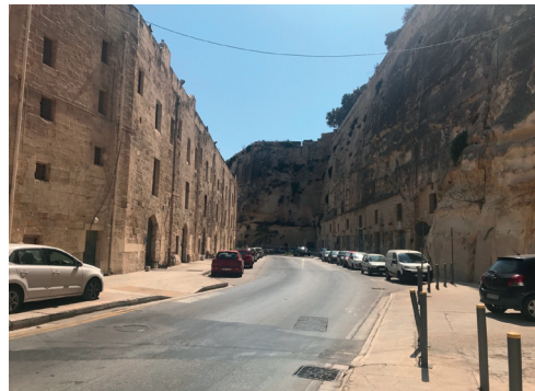
(b) View of the road created behind Pinto Stores which caused the demolition of the backyards to Pinto Stores
