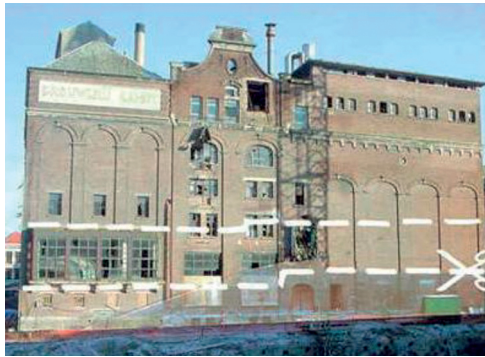
(a) Before rehabilitation/reconstruction
