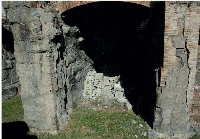
Figure 4.8. The restoration of the 1970s in Roman Theatre, Teramo, Italy did not consider that modern bricks integrating gypsum-sandstone blocks were too heavy and would detach, © L. Migliorati.
