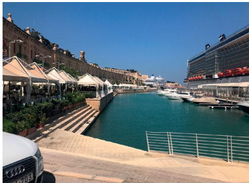
(a) Pinto Stores severed from their original context and direct link with Valletta Grand Harbour due to the marina which serves as a cruise liner terminal
