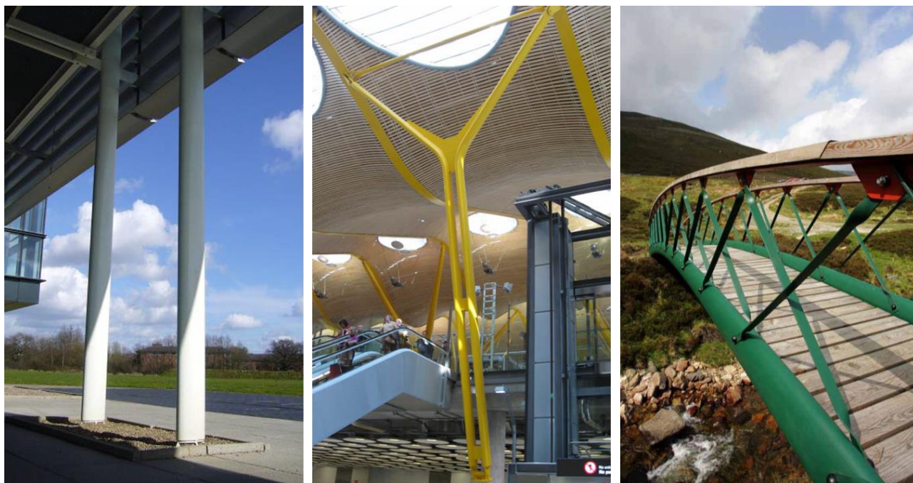
Slika 1. Primeri primene EHS preseka [6]: (a) objekat Ziman; (b) aerodrom Barajas; (c) pešački most u Škotskoj Figure 1. Examples of EHS application [6]: (a) Zeeman building; (b) Barajas airport building; (c) pedestrian bridge in Scotland
