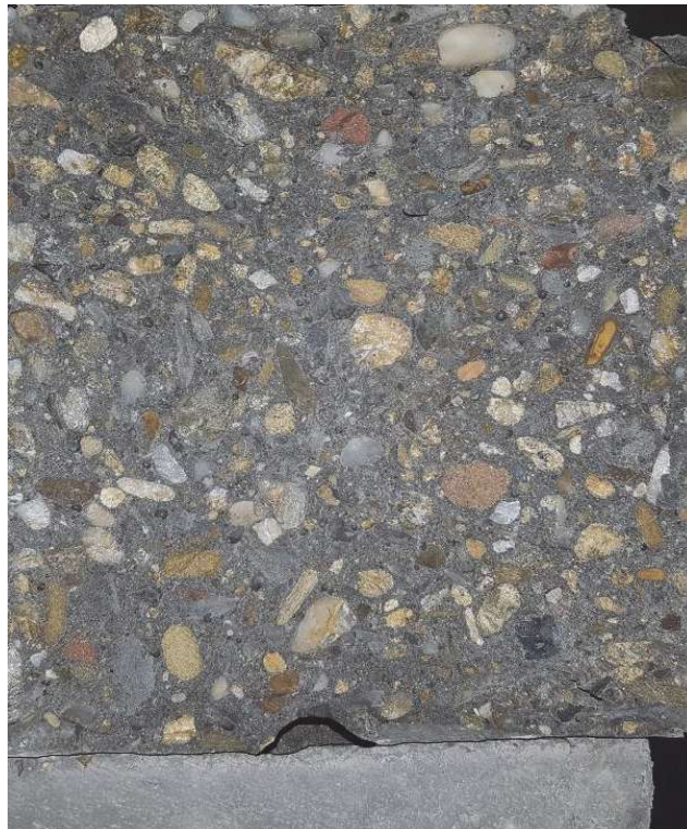
Figure 9. Appearance of the sample after the splitting for water penetration measurement
