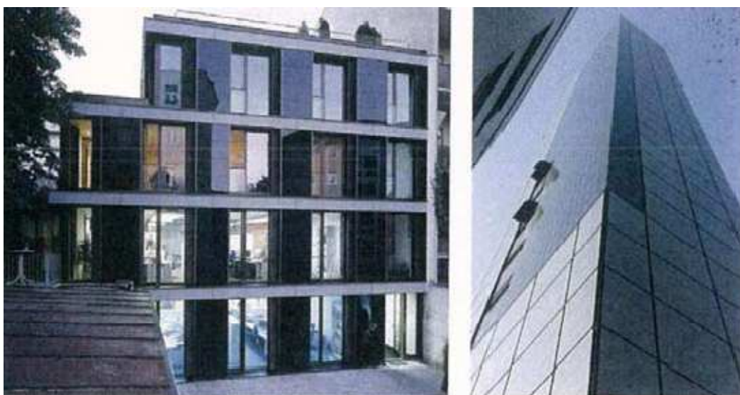
Figure 6. Facade systems with CIS modules based on copper indium disulphide
