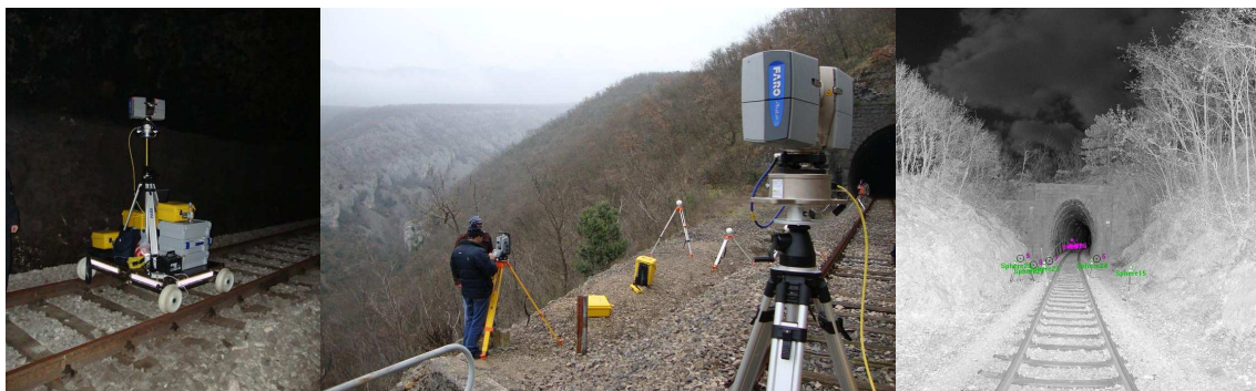
Figure 3: Scanner mounted on the cart and spheres on the tripods
