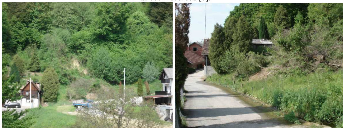
Figure 4: In the spring of 2008 a new landslide in Vidovec was created. Landslide is located within the route of the main faults of the Zagreb fault zone. In the overlying wing of the cliffs there is a fault in the relief. Due to tectonic activity there was a cliff destabilization and the activation of landslides [7].
