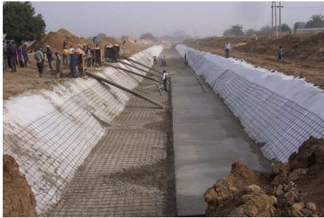
Picture 12: Canal construction
