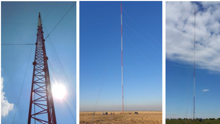
Figure 1 - Installed guyed masts of 120.78m, 160.00m and 126.30m height, respectively (source: NETInvest Engineering and Consulting Solutions)
