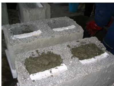
(a) Punjenje blokova svežim betonom Filling with fresh concrete
