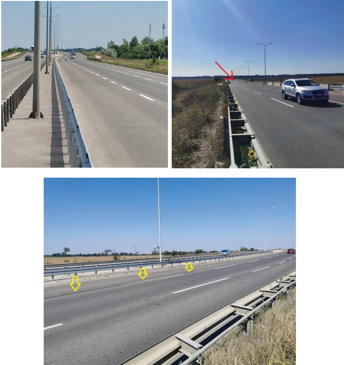
Figure 4. Road deviation at the location of future at-grade intersection area
