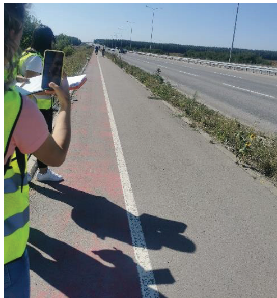
Figure 7. Inadequate bicycle path width
