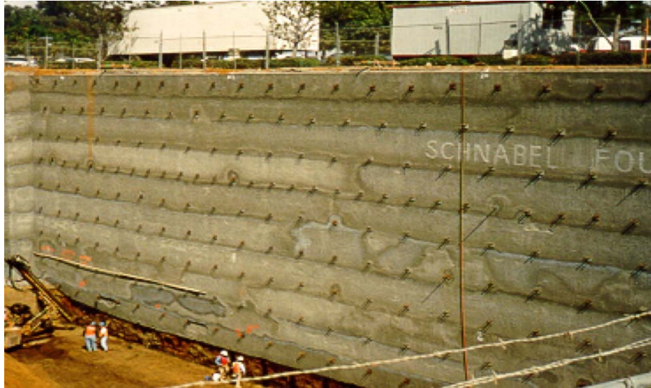
Figure 3. Anchoring of the support structure
