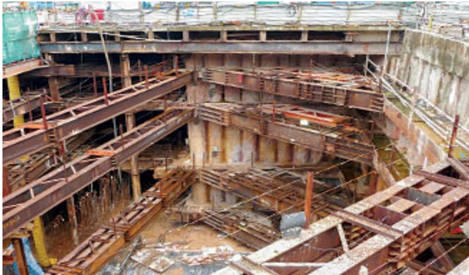
Figure 2. Shoring of the support structure
