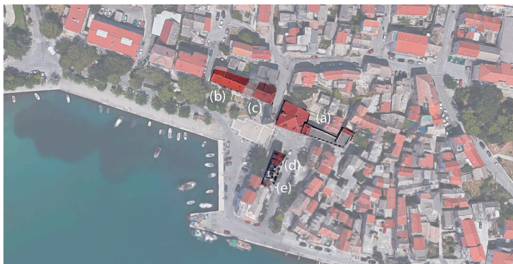
Figure 7. A view of Kaštela case study site and the five buildings analysed.
