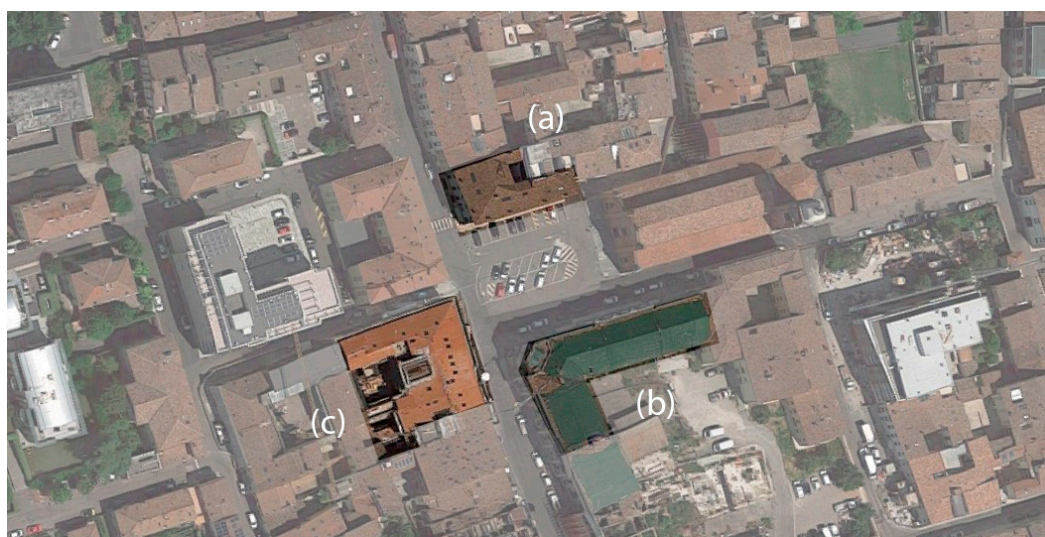
Figure 5. A view of the Mirandola case study site and the three buildings analysed.
