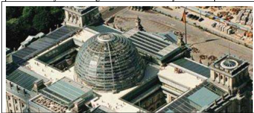
Fig. 4: Solar panels at the Reichstag building in Berlin [3]
