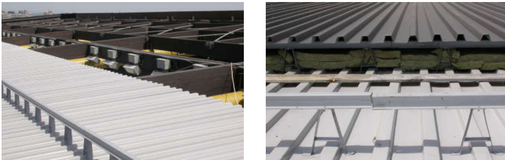
Figure 7: New roof cladding positioning.
