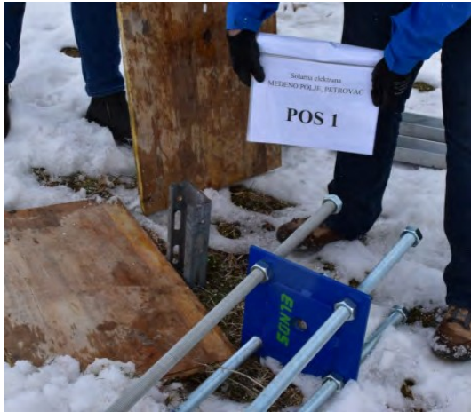
Figure 6: The appearance of the anchor POS 1 before testing
