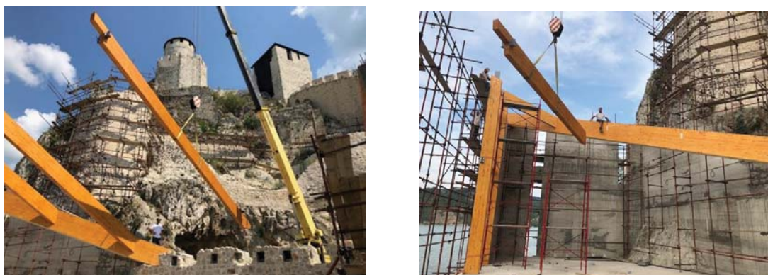
Fig. 9. Assembly of glued laminated roof structure
