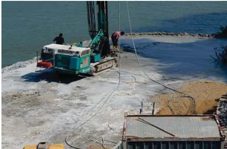
Fig. 6. Execution of jet grouting columns
