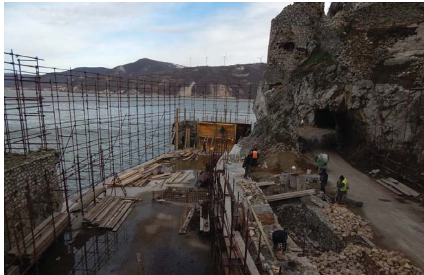
Fig. 8. Commencement of work on the above-ground part of the structure
