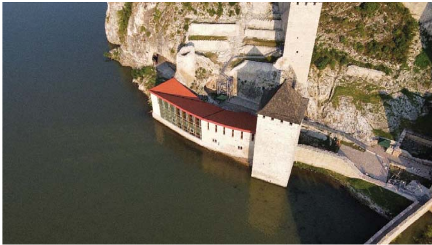
Fig. 14. The Palace after reconstruction
