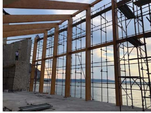
Fig. 10. Assembly of glued laminated roof structure
