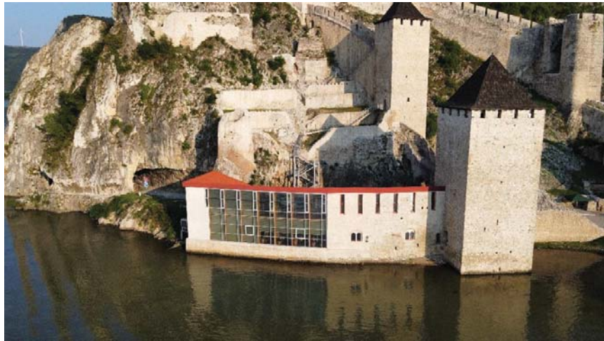
Fig. 13. The Palace after reconstruction
