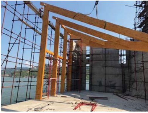
Fig. 10. Assembly of glued laminated roof structure
