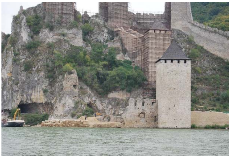
Fig. 12. The Palace before reconstruction
