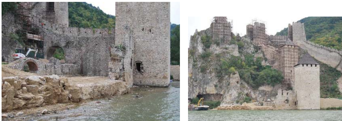
Fig. 7. The Palace foundations after jet grouting repair
