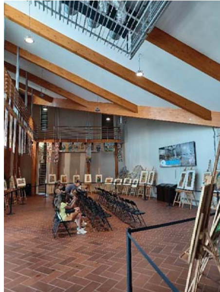
Fig. 11. Current interior of the Palace. Left, traditional timber structure; right, modern glued laminated timber structure
