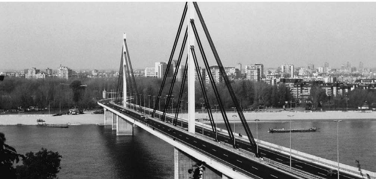
Fig. 19 The "Sloboda" roadway bridge over the River Danube in Novi Sad - after reconstruction
