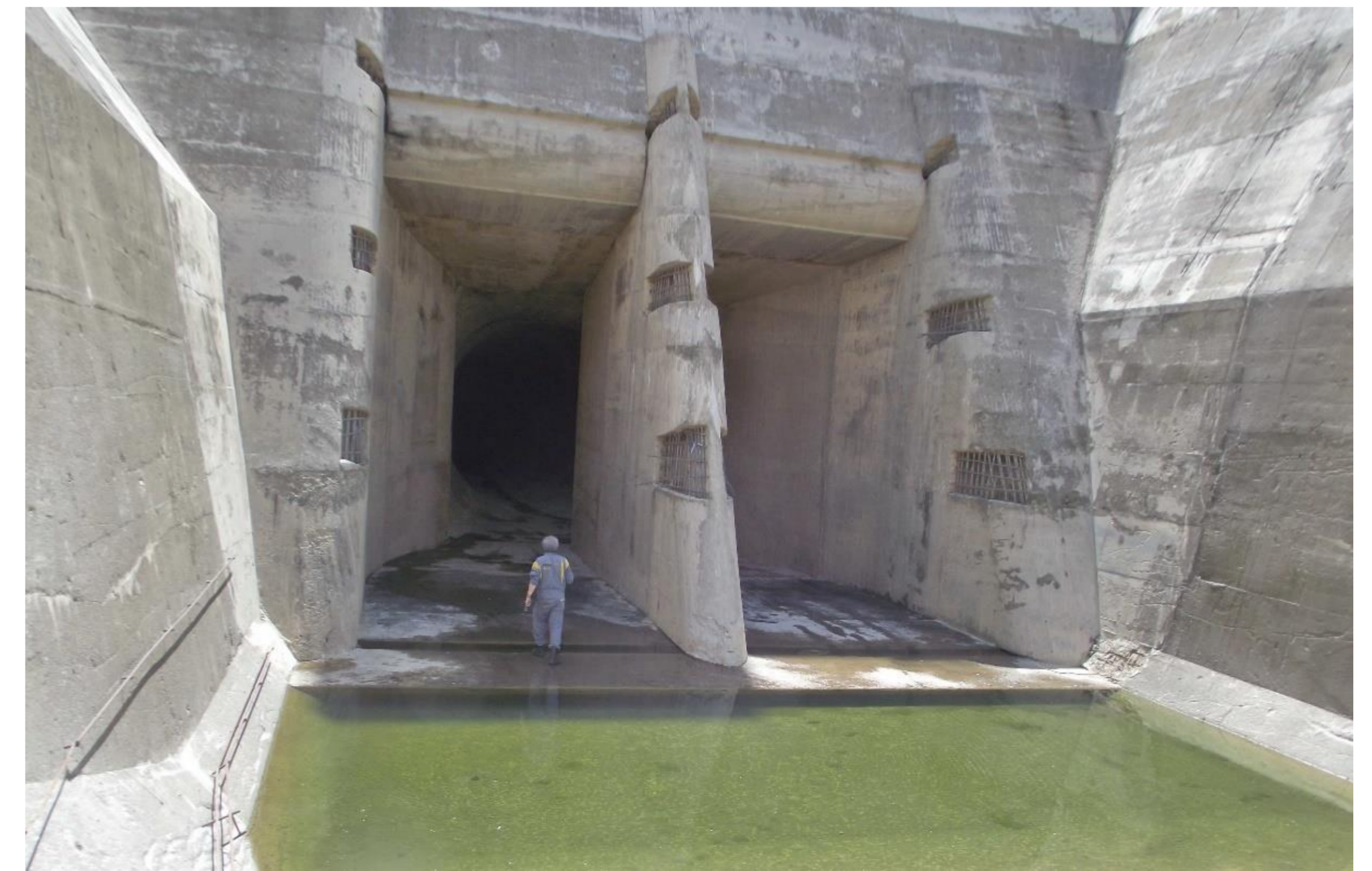
Figure 2. Entrance to the derivational tunnel
