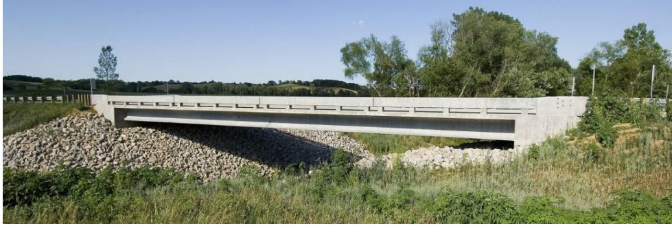
Figure 5. Mars Hill Bridge, Iowa, USA (2006) [20]
