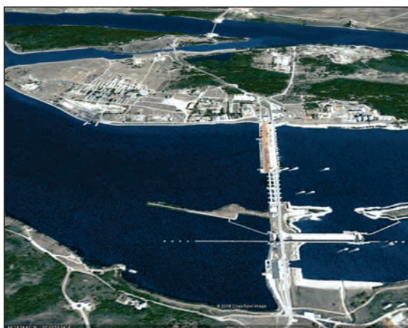
Figure 21. Iron Gate 2 (Djerdap 2) hydropower plant (taken from Google Earth, 2009; location: 44°18'24.61” N/22°33'53.54” E)
