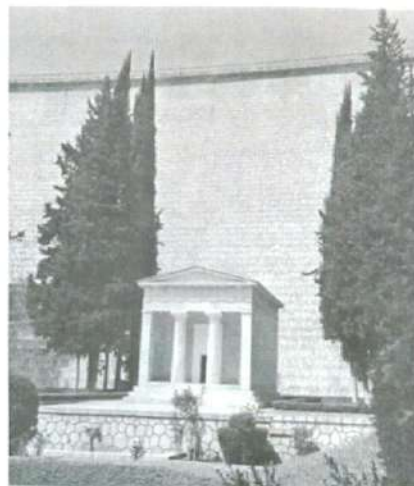
Figure 3. Marathon dam for water supply of Athens
