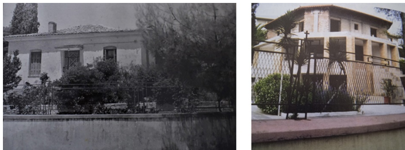
Figure 10. Old and new presbytery next to the St. Luke church [23]
