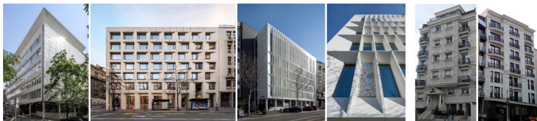
Figure 7. Renovation of facades on the existing three office buildings (Authors: Remorker Architects, 2018-2019) (left) and „Starletarchitecture“ (eclectic manner and bad tendency) (right)
