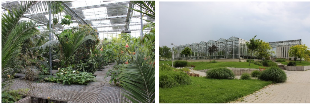
Figure 5. Figure 5. South Pest Wastewater treatment facility (Budapest, 2012, architecture authorship unknown to us): Plants grown in controlled environment assist in the process of aerobic/oxygenated fixed-film waste water treatment.) Photo: paper's first author
