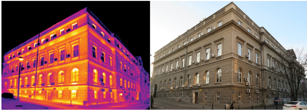
Figure 3. Thermal imaging and photograph of the street facade of the building of the City Municipality of Zemun. Heat losses are evident in the area where concrete beams are - over windows and in the area of window openings
