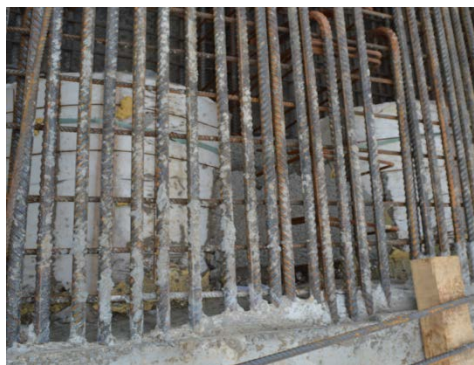
Figure 9. Deck slab reinforcement
