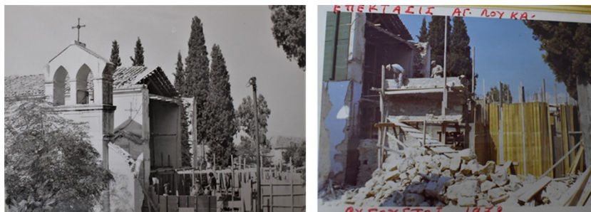
Figure 8. Construction works at the St. Luke church in 1972 [23]
