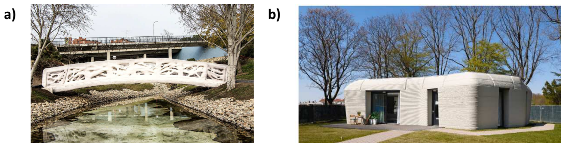
Figure 4 - Representative example of using 3D printing technology in concrete structures: a) bridge in Madrid, Spain, b) Milestone House
