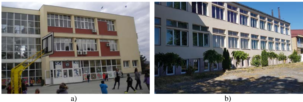
Figure 9 – Infilled RC frame schools in Serbia: a) Primary School Sveti Sava in Mladenovac and b) Primary School Slavko Rodić in Sečanj
