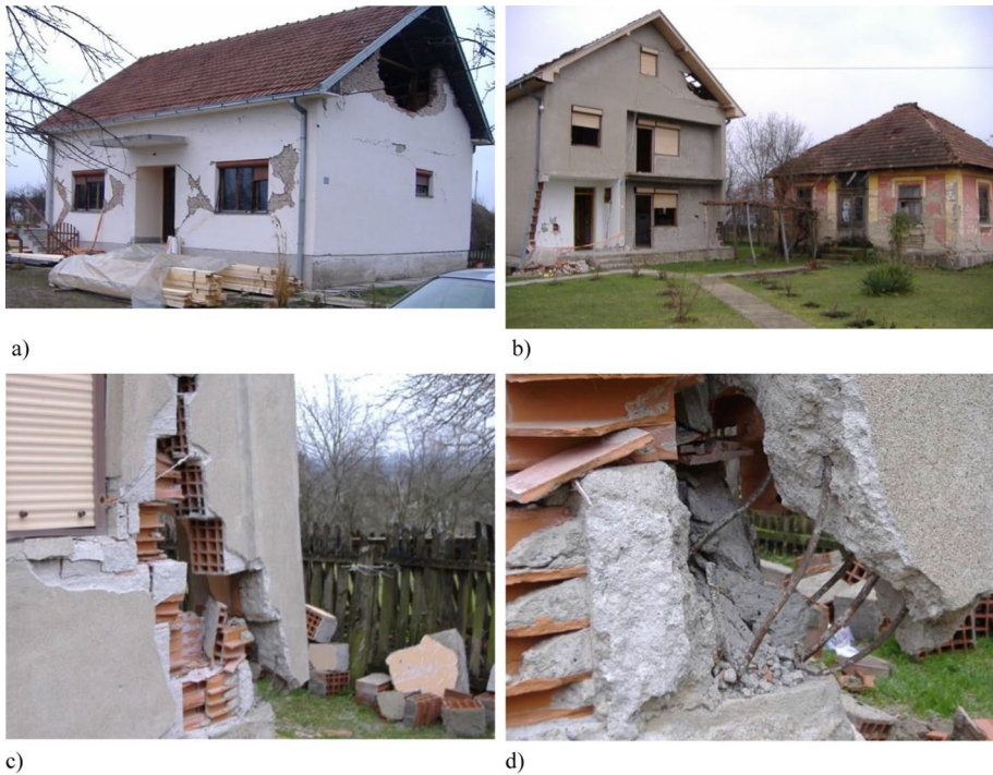
Fig. 28 Rural single-family masonry buildings affected by the 2010 Kraljevo, Serbia earthquake: a a severely damaged type M2 building; b a damaged inadequately confined M4 type building (left) adjacent to an undamaged old timber-frame (bondruk) building; c and d damage at the corners of the building shown in figure b due to construction flaws (Manić and Bulajić 2014)
