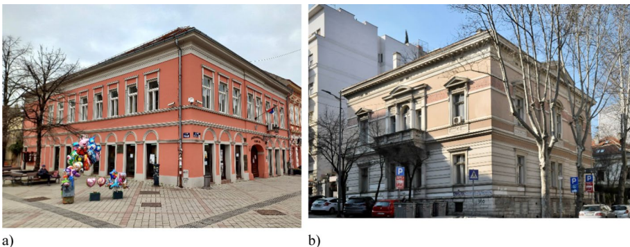
Fig. 10 URM buildings with flexible diaphragms: a type M1: an URM building with adobe walls constructed at the beginning of the nineteenth century in Dunavska Street 2, Novi Sad and b Type M2: an URM house with brick masonry walls constructed in Belgrade in 1884
