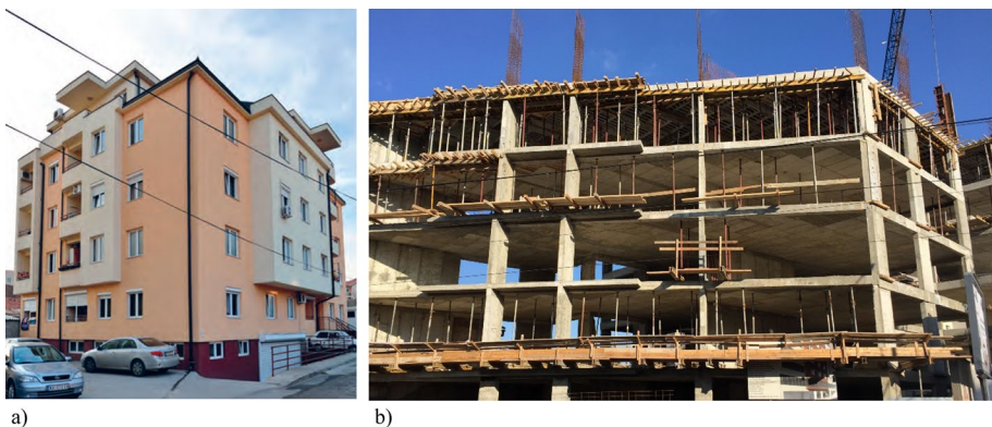
Fig. 14 Cast-in-situ RC frame-wall building typology—type RC2: a a 4-storey multi-family residential building in Belgrade (Jovanović Popović et al. 2013c) and b an RC2 building under construction in Belgrade
