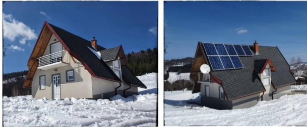
Figure 1. Exterior view of the weekend cottage in Kriva Reka, Kopaonik
