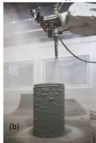
Fig. 2. 3D concrete printing using the spraying method (SC3DP). [5]
