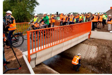
Fig. 5. Pedestrian bridge over the Peelse Loop canal [10]
