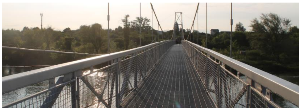
Figure 1. Suspension footbridge over the Vrbas river in Banja Luka (Priječani sub-area)
