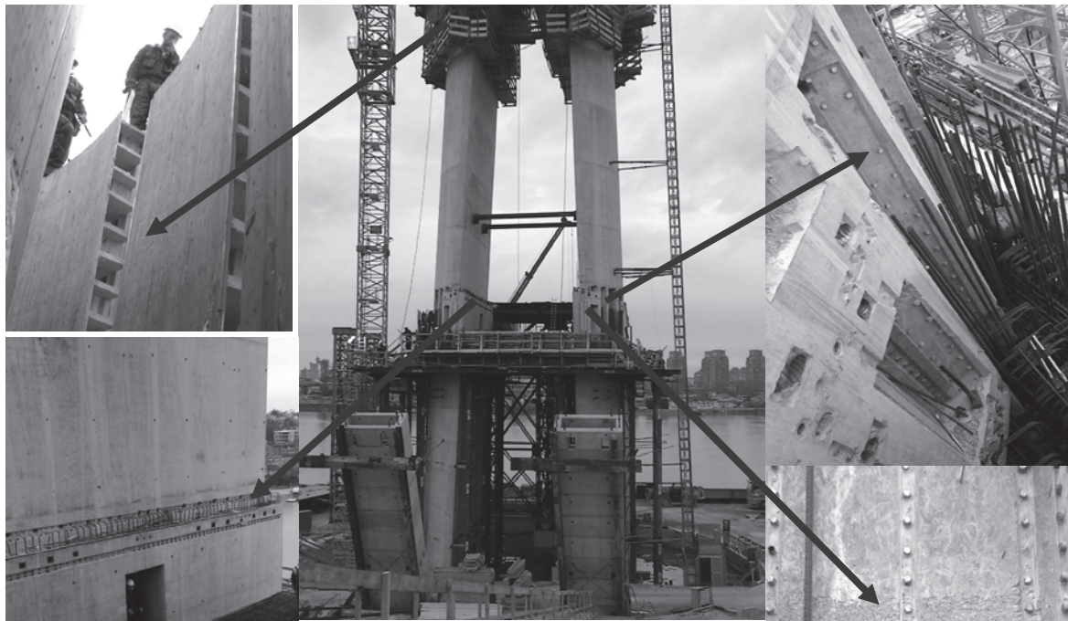
Slika 6. Primena mehaničkih spojnika – Most preko Ade u Beogradu Figure 6. Rebar Couplers Application – Ada Bridge in Belgrade
