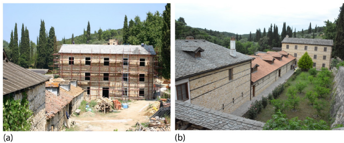
Figure 1. The Haybarn Complex: Mulekeepers' House, Stable, Haybarn (from left to right): (a) former appearance, (b) after the restoration (photos taken by the author)
