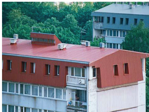
Figure 2. Typical building with attic annex.
