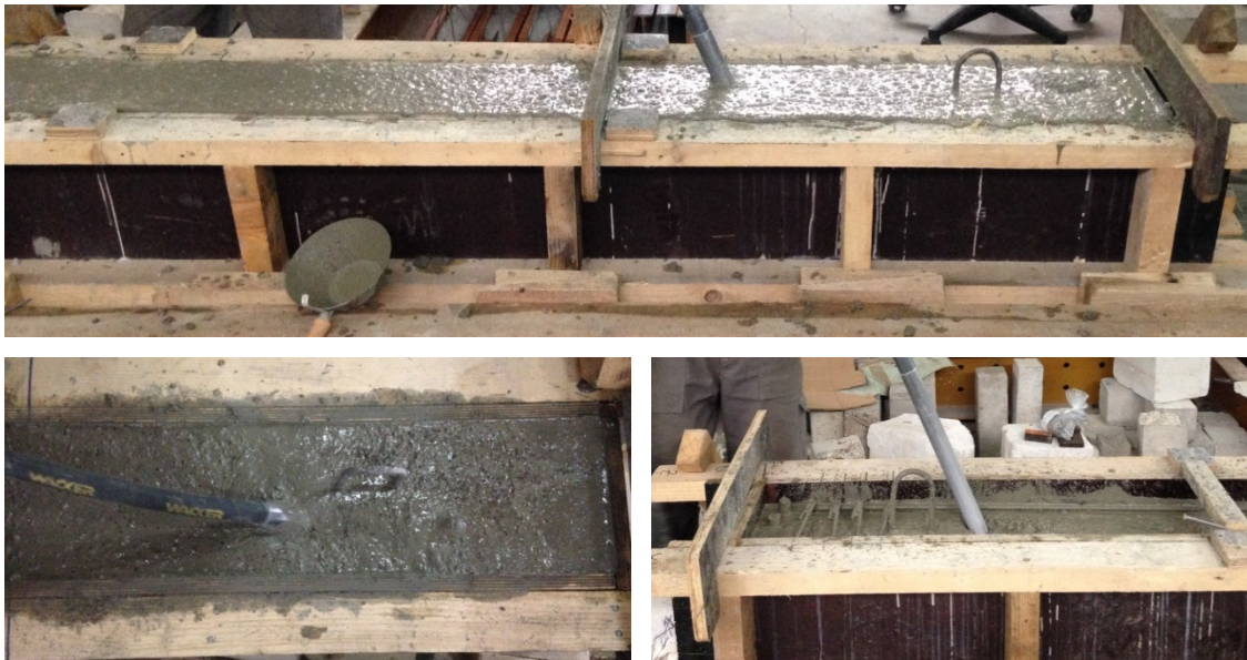
Figure 4. 11 Concrete casting and vibration
