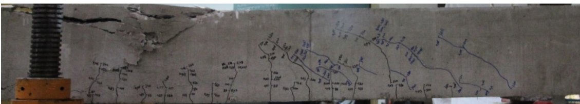
Figure 4.192 Crack pattern in the back side of the OPC-3 beam after failure
