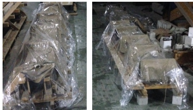
Figure 4. 12 Curing of the beams
