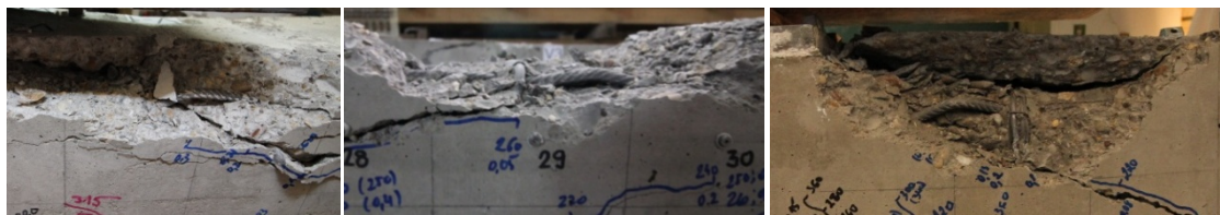
Figure 4.190 Buckling of the compressed reinforcement at failure in the OPC-2, HVFAC-2, and HVFAC-3 beams
