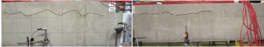
Figure 4.39 Longitudinal cracks in HVFAC beams prior to loading
