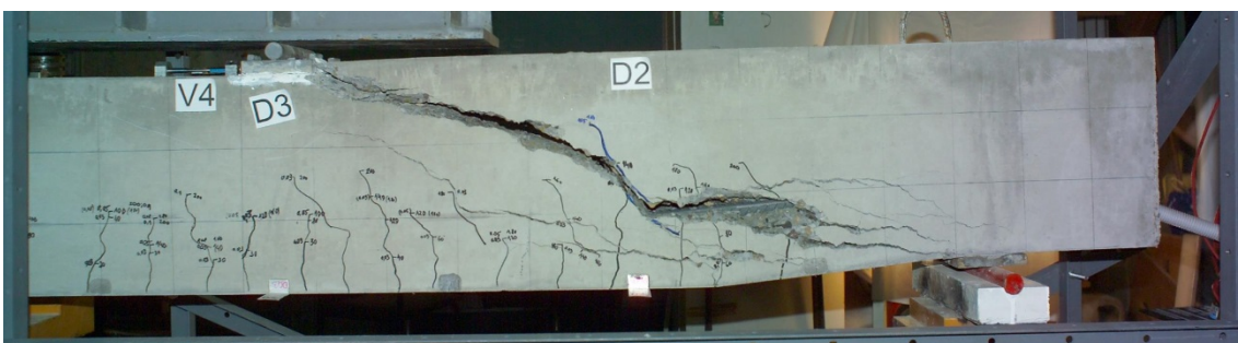
Figure 4.168 HVFAC-1 beam failure crack pattern
