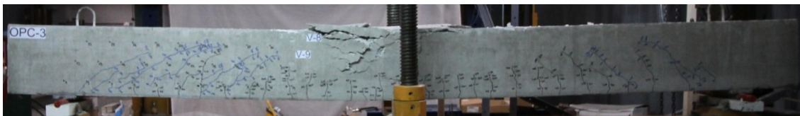
Figure 4.191 Crack pattern in the front side of the OPC-3 beam after failure
