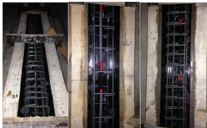
Figure 4.9 Reinforcement of beams tested in flexure in formwork
