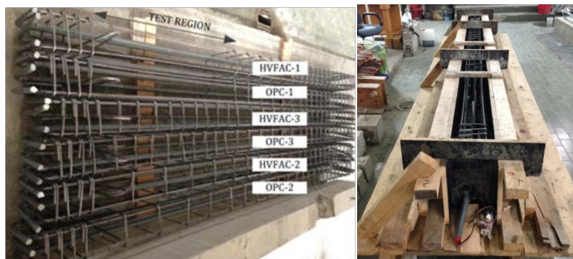
Figure 4.149 a) Reinforcement of beams tested in shear and b) beams' formwork
