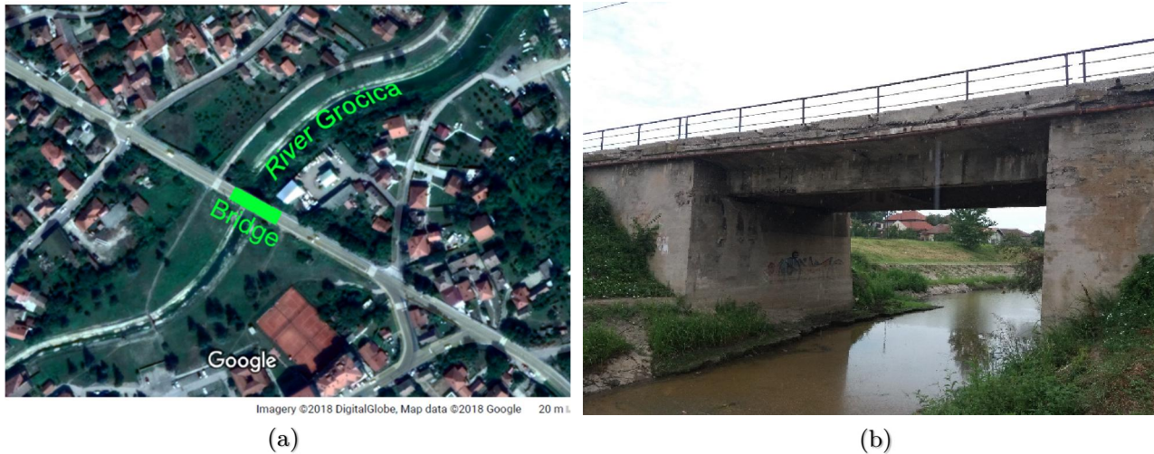
Figure 5.1. Case study: Bridge over river Gročica, located in Grocka municipality of the city of Belgrade, Serbia. (a) Aerial photograph showing the location of the bridge, and (b) Perspective view of the bridge.
