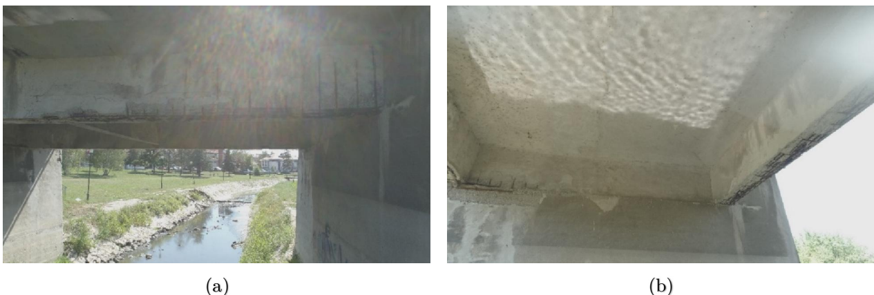
Figure 5.5. (a) Oversaturated photo of the bridge, (b) water reflection on the bridge deck.
