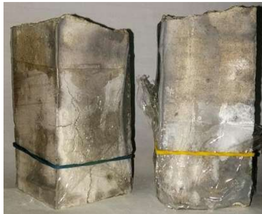
Figure 6 – Cracks on the sides of the 1/1-30 mortar samples
