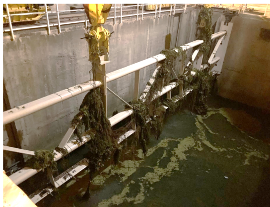
Figure 6. Vegetation build-up on the steel frame during the measurements
