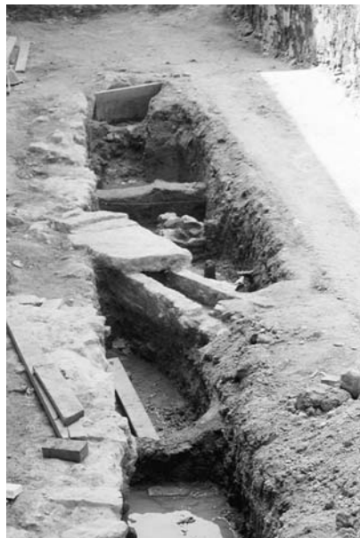
Fig. 3. – Turkish drain made of stone slabs
