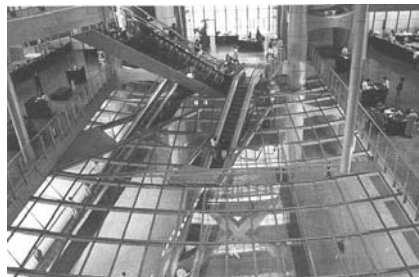
Slika 2. Hong Kong Shanghai Bank, Hong Kong, China; Norman Foster & Partners
