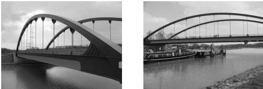
Figure 3. Bridge over the Dortmund-Ems channel, Muenster Hilstrup, Germany
