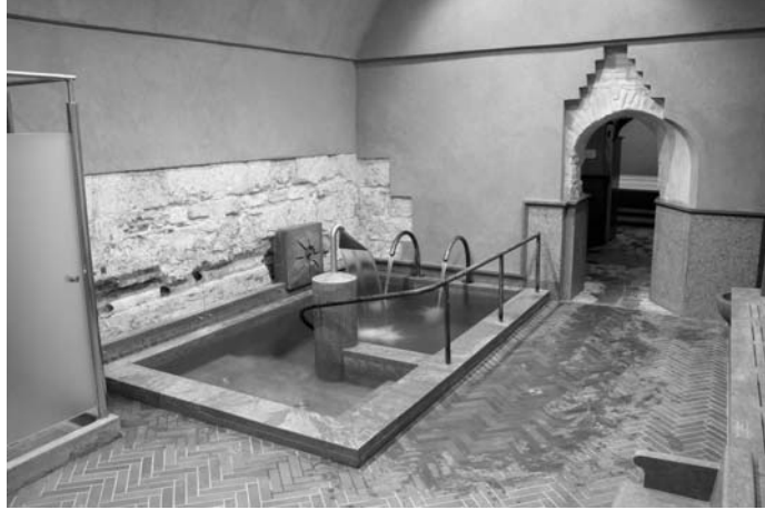
Fig. 8 - Small basin, Turkish water-pipe system in the wall
