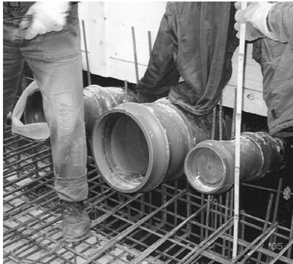
Fig. 5 - Reinforced concrete wall against the flood
