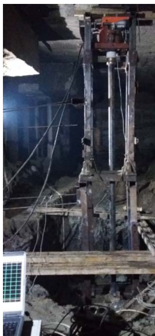
Fig.1. Set for sample testing with hydraulic presses
