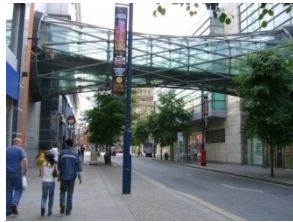
Fig.2 Hyperboloid bridge in Manchester
