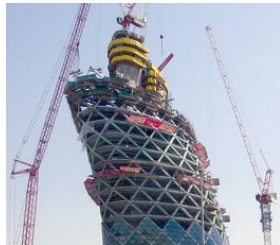
Fig. 4 Capital gate in Abu Dhabi
