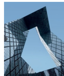
Fig.6 CCTV in Beijing
