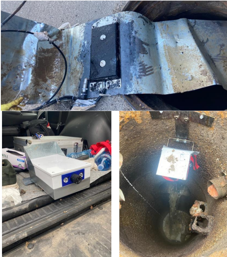
Slika 4. Gore) Elektromagnetni sensor na nosećem limu nakon demontaže; Levo) Kamera pre montaže; Desno) Montirana kamera na mernom mestu Figure 5 Above: Electromagnetic flat sensor on metal sheet support after deinstallation. Bottom left: NIR camera before installation, Bottom right: NIR camera in installed position
