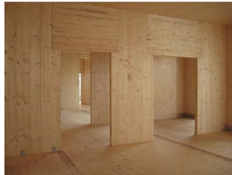
Fig. 2. CLT panels as wall and floor elements
