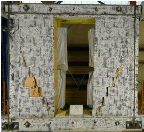
Figure 7. Damage to masonry infill at 1.2 % of in-plane drift
