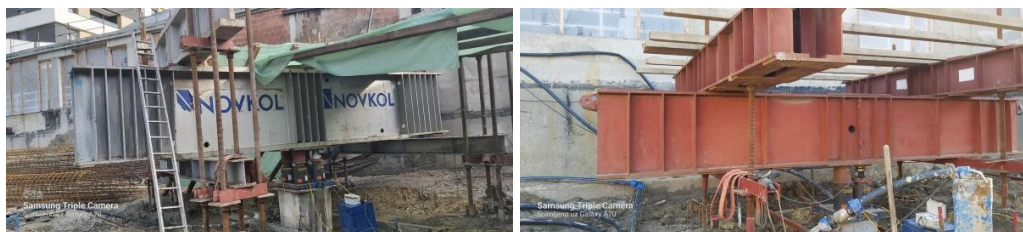
Figure 4. Photos on-site installations of testing piles T1 (left) and T2 (right)
