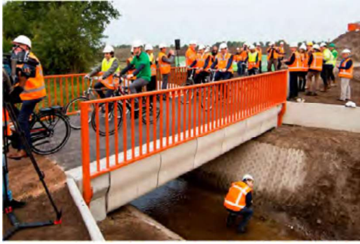
Figure 6. Pedestrian bridge over the Peelse Loop canal [10]
