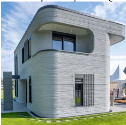
Figure 4. First-ever 3D printed concrete house in Germany (Beckum House) [8]
