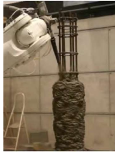
Figure 2. 3D concrete printing using the spraying method (SC3DP). [5]
