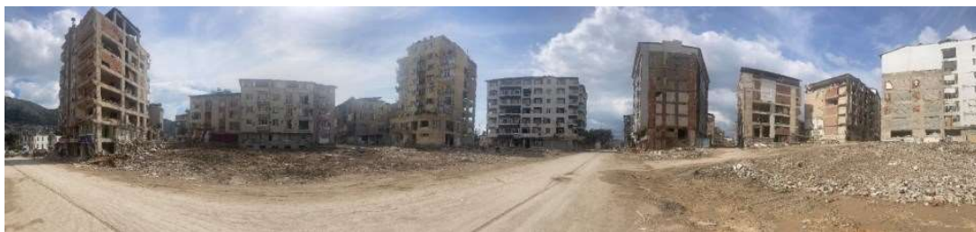
Diagram 4. Ruins of Antakya (province Hatay), showing the prevalence of RC buildings (credit: SUZI-SAE).)
