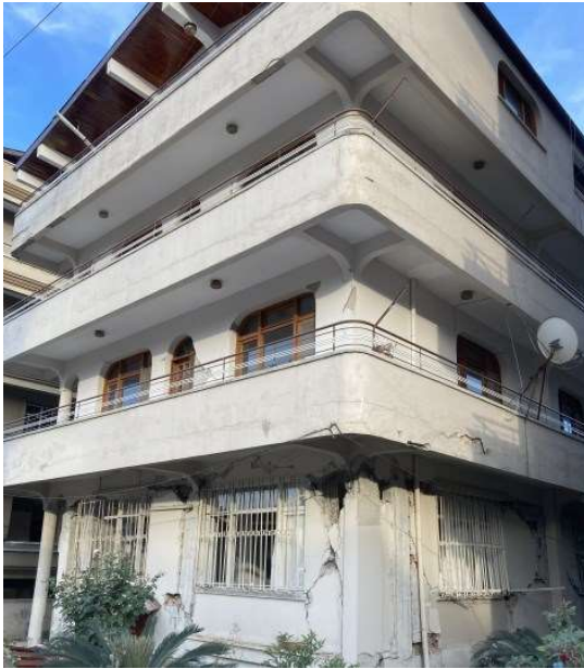
Diagram 16. Damage of an RC column without ties in the critical zone at the top of the first floor level, a low-rise residential building in Antakya (Hatay)
