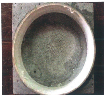
Figure 5: Surface of concrete sample after 25 cycles of freeze-thaw and salt attack [7]
