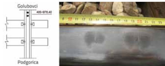
Figure 8. Multiple squat defect (typically shaped as "lungs")
