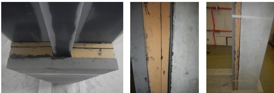
Figure 3.8 Placing U-shaped elastomers at the columns and top beam of the RC frame
