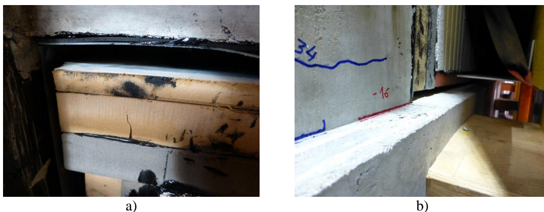
Figure 5.79 a) Gap formation in the corner of the frame and b) uplift of the wall base
