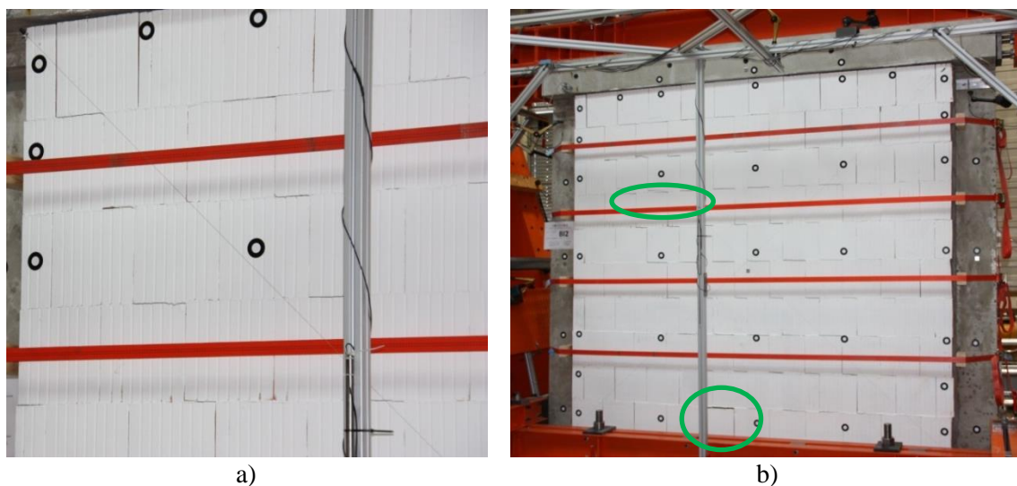
Figure 5.31 a) Opening of bed joints and b) stepwise cracks in compressed diagonal and cracks in the bricks
