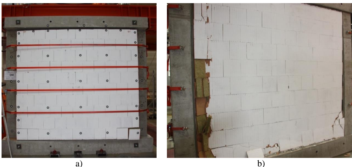
Figure 5.68 a) Front view and b) damage of the masonry wall on the backside at the end of the test CIO
