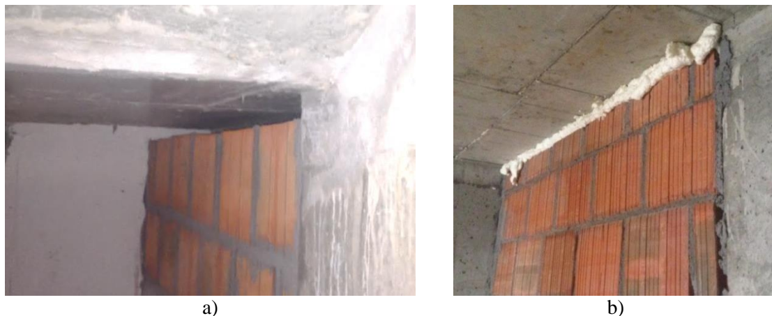
Figure 2.18 Gap at the top a) before and b) after filling with polyurethane foam
