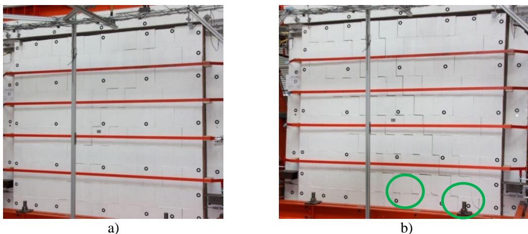
Figure 5.58 a) Formation of stairstep cracks and b) cracks in the blocks at 2.1% of drift
