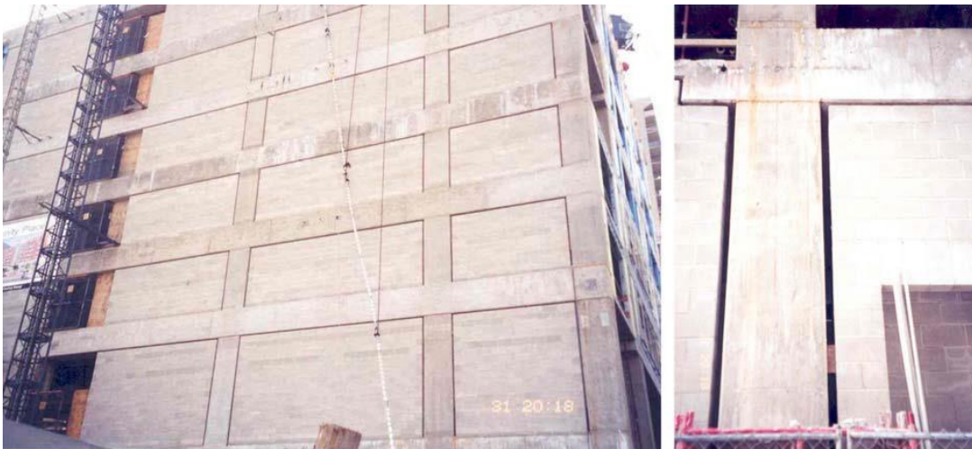
Figure 2.24 Isolated infill walls from RC frame with gaps (Aliaari and Memari, 2005)
