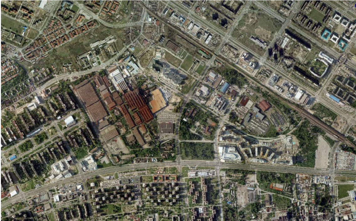
Figure 4: An example of dilapidated industrial complex located between residential blocks – New Belgrade (Geosrbia)
