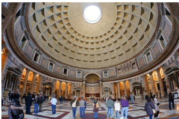
Figure 4. Example of coffered dome in Pantheon, Rome constructed at the beginning of a new era – a question for all of us, were those builders, in terms of the durability of their buildings, smarter and more competent than today's builders, whose buildings from the modern concrete look very bad even after less than two hundred years [16]
