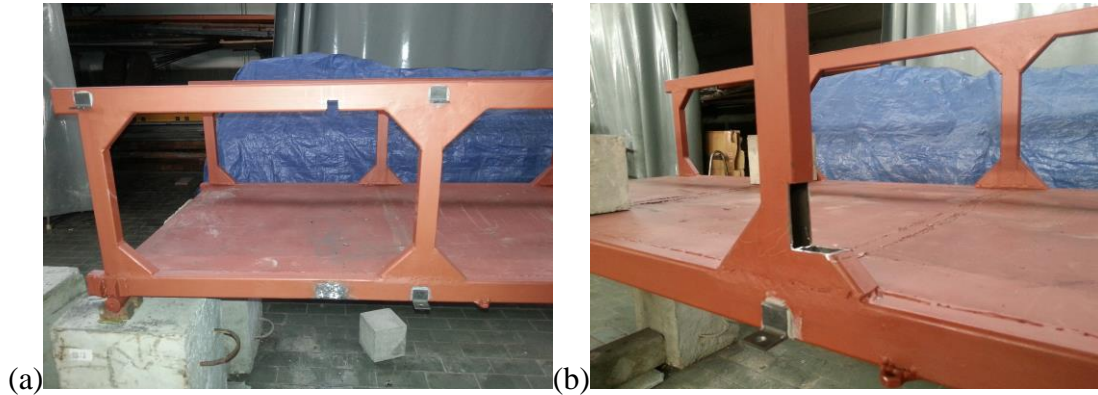
Figure 5.43. Extent of damage scenarios in DC-1 and DC-2 of the damaged Vierendeel bridge model
