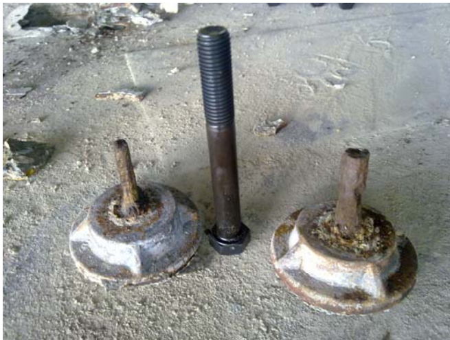
Figure 4. Comparison of the original corroded bolts with the new bolt of the same diameter.
