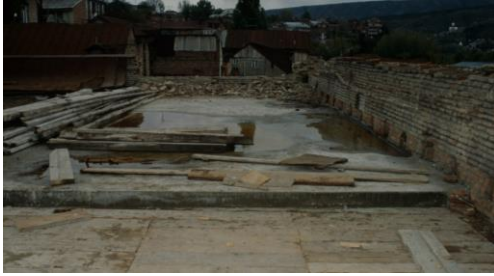
Figure 8. Timber-concrete composite floors: Strengthening of wooden floors with cast in place RC in Tbilisi, Georgia
