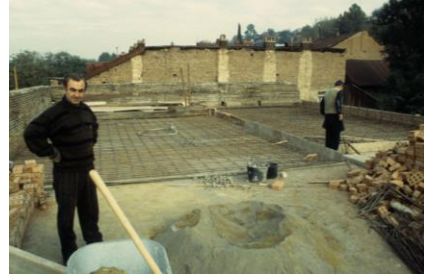
Figure 8. Timber-concrete composite floors: Strengthening of wooden floors with cast in place RC in Tbilisi, Georgia
